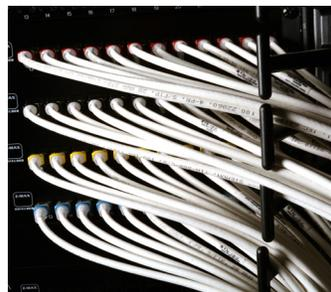
Smaller diameter cable significantly reduces bundle and pathway fill for space savings.
